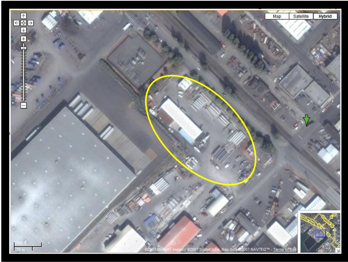
Figure 2 Overhead View of the Ershigs C Street Facility
